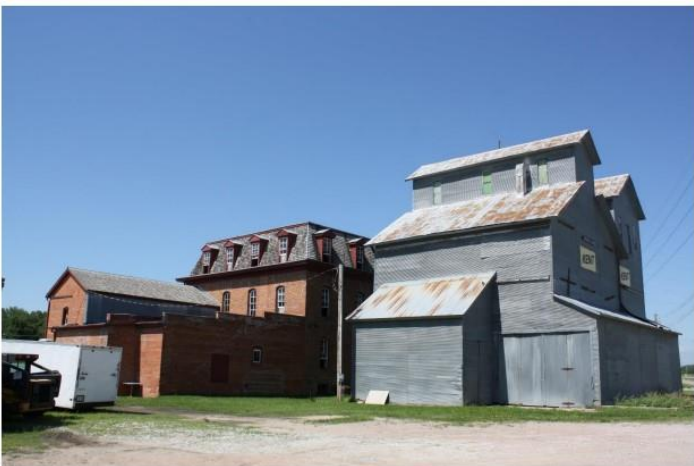
8. View of elevators and mill looking southwest.
