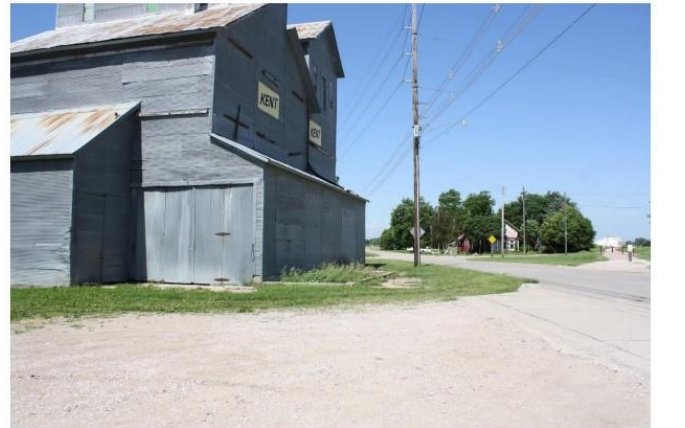
10. View showing elevators at left and Cowboy Trail at right looking northwest.
