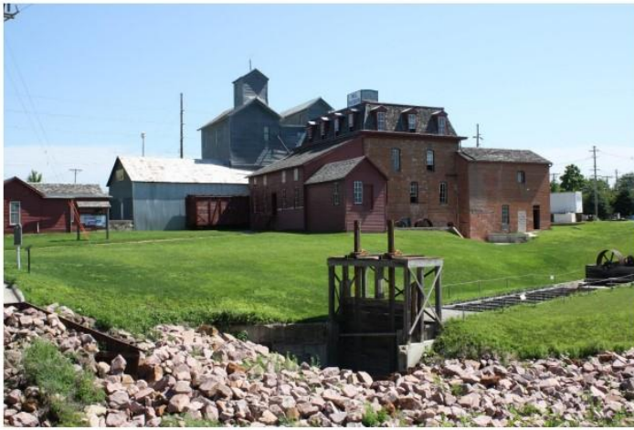
1. View of mill and elevators looking northeast
