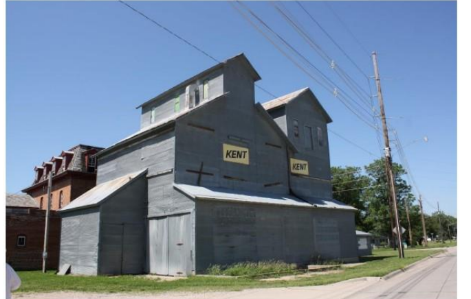
6. View of elevators looking southwest.
