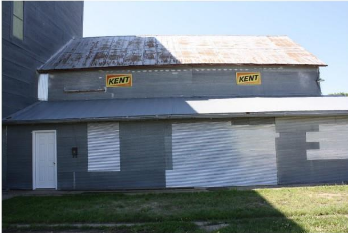
5. View of elevators looking south.
