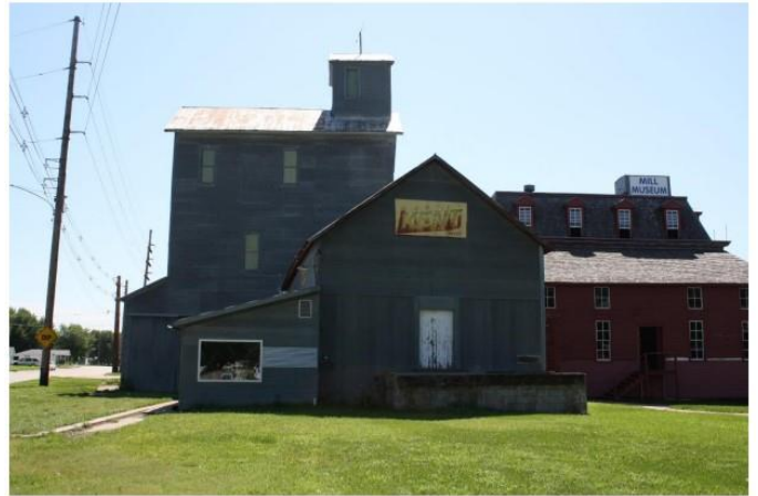
4. View of main mill building and elevators looking east.
